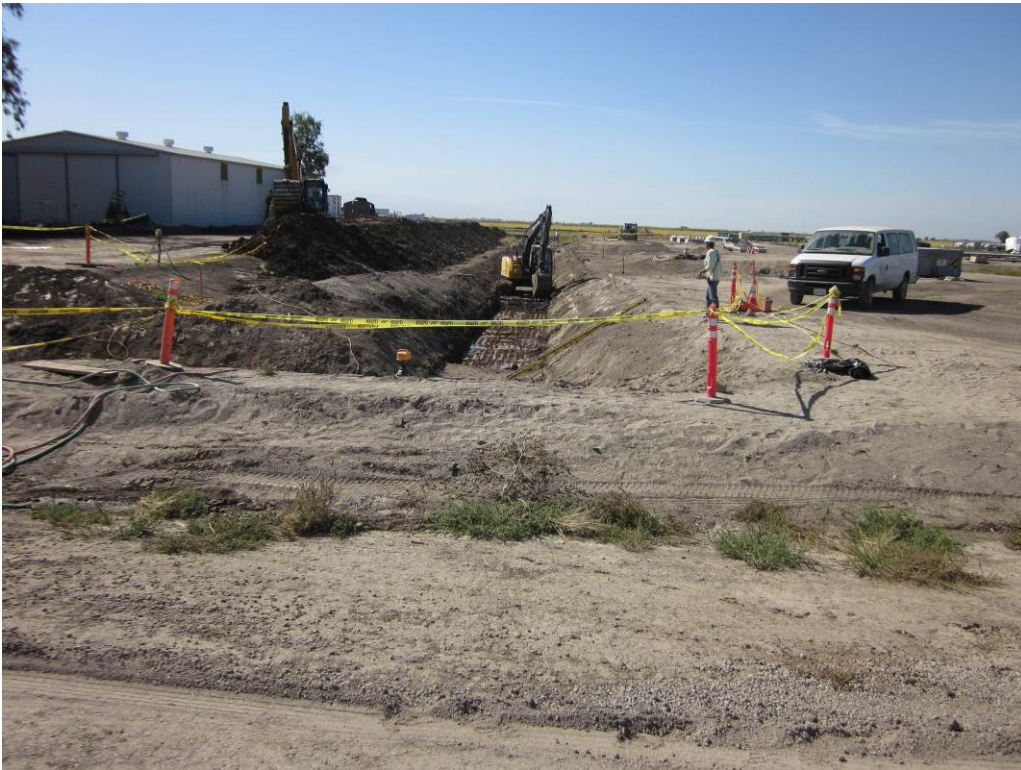
Photo 2: Trench excavation at the south end of the Compressor Station site.
