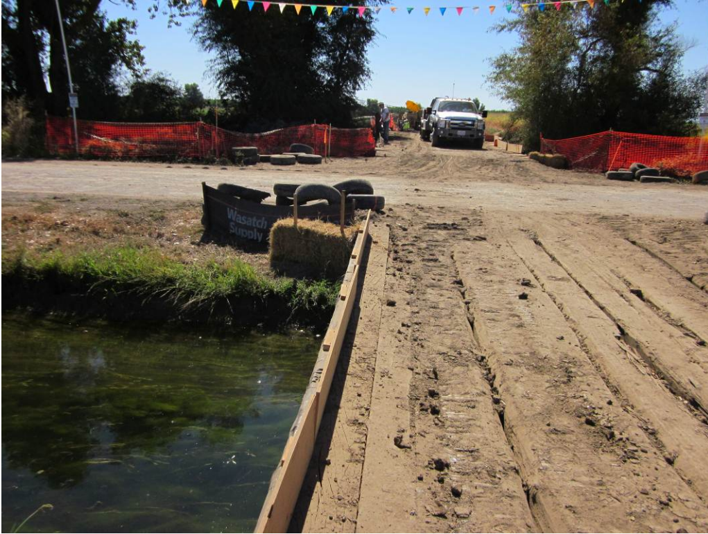
Photo 3: Sensitive resource exclusion fencing and temporary bridges at D-5 and D-6.
