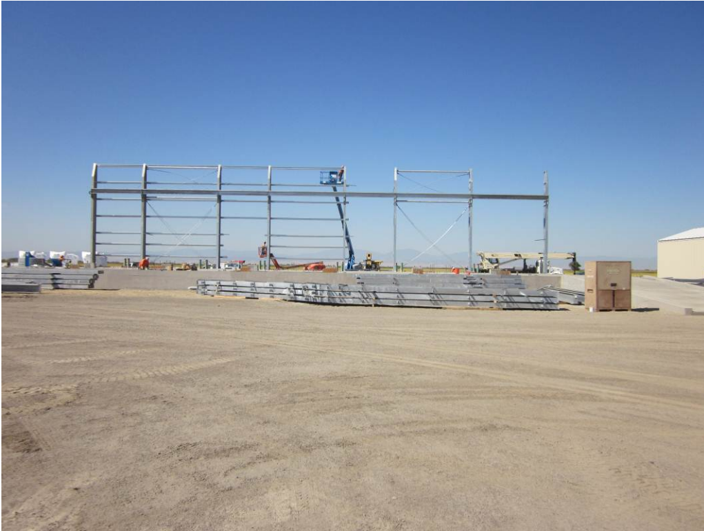
Photo 1: Framing of compressor building at the Compressor Station site.
