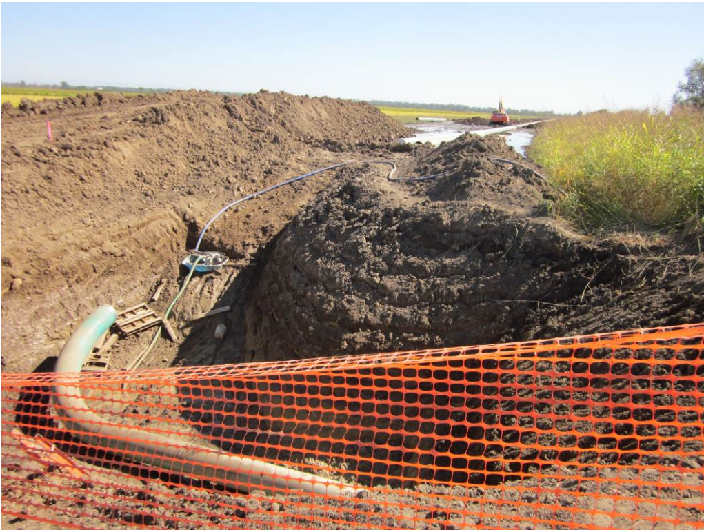
Photo 4: Auger bore hole and dewatering activity at D-10a.
